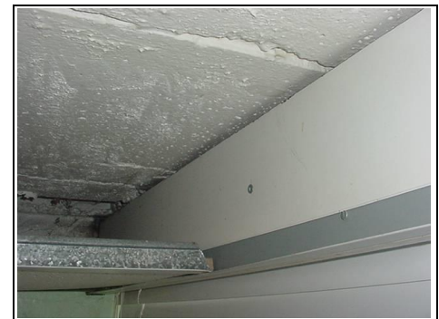
Within ceiling void
