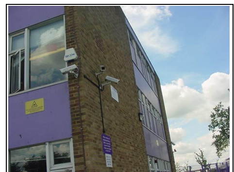
Cross wall construction
