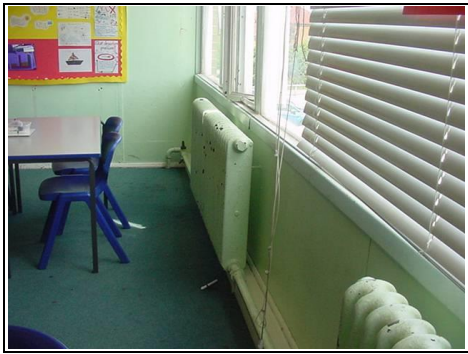
Lower wall and radiator
