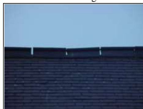
Overview of slipped slate to the south elevation
