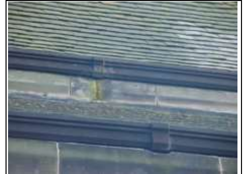
Leaking gutter sitting on a wall.
