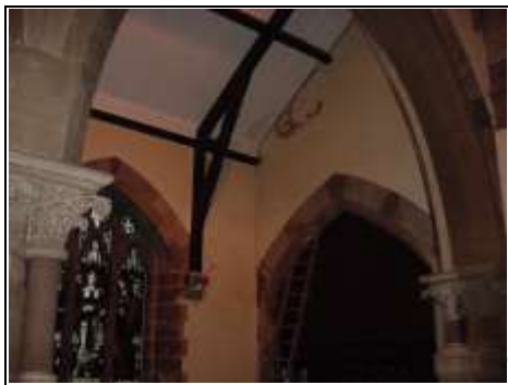
High level dampness to the Vestry side of the church
