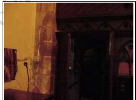
Low level dampness to the north aisle
