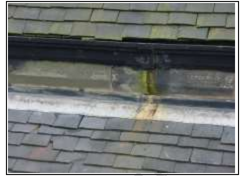
Leaking gutter
