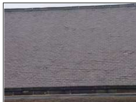
Close up of ridge, needs re-bedding
