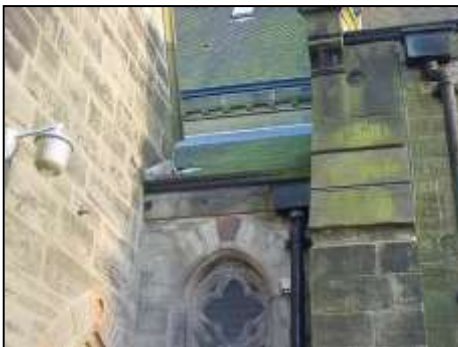
Overflowing valley gutter to north door entrance
