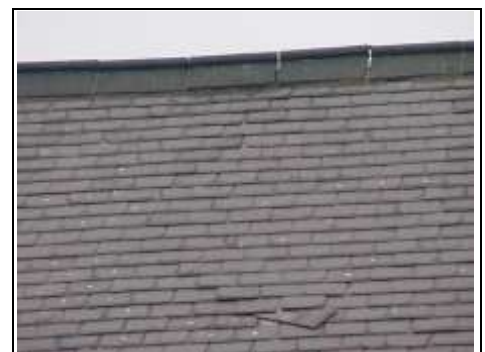
Slipped slates and deteriorating ridge tiles.
