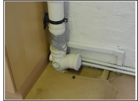
DIY repairs to soil and vent pipe
