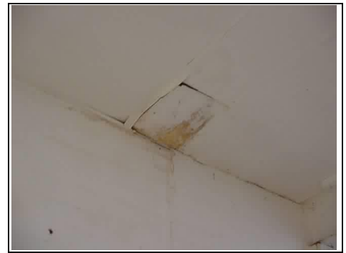
Roof leaks
