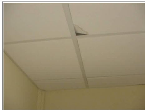
Broken ceiling tile in computer room
