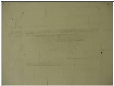
Pattern staining in open plan office
