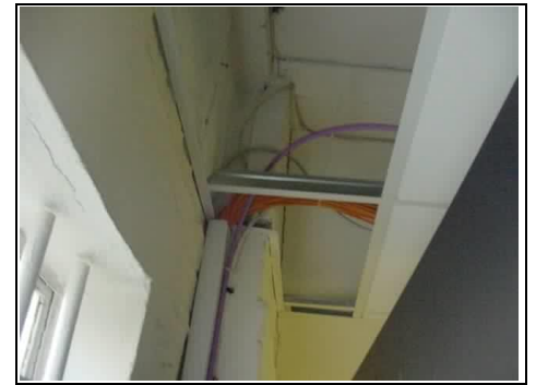
Missing tiles in ceiling in computer room
