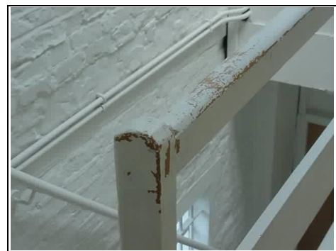
Close up of worn hand rail
