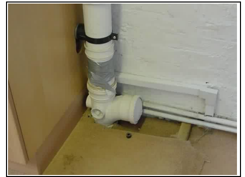
DIY repair to soil and vent pipe
