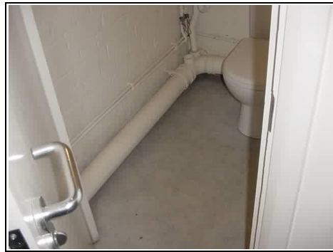
Soil and vent pipe needs cleaning and painting
