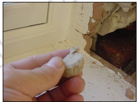
Saturated plasterboard to the reveal of the window
