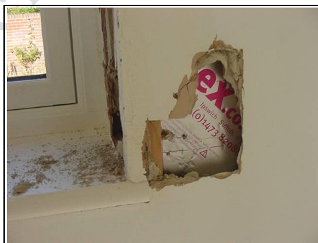
Celotex insulation board visible to the wall side of the window
