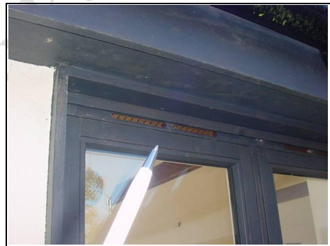
Trickle vent in window
