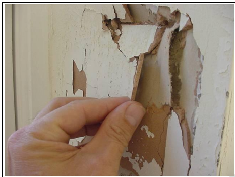
Skim coat of plaster that's been put on top of plasterboard. This is saturated.
