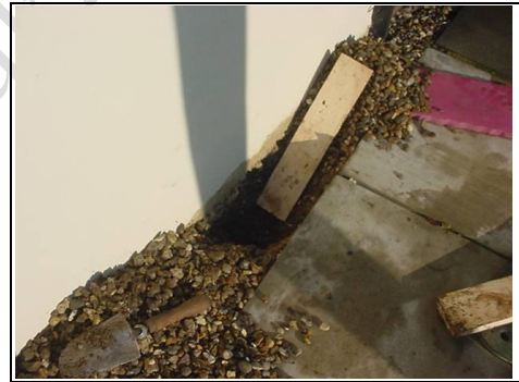
French drain (rear) dug-up approximately 100mm deep
