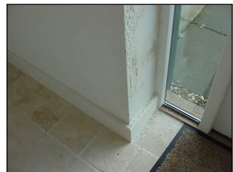
Reveals to the rear wall are flaking
