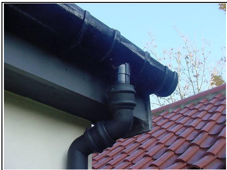
Guttering to downpipe needs to be checked it is watertight.
