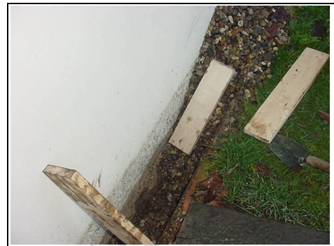
French drain (front) dug –up to approximately 150mm deep
