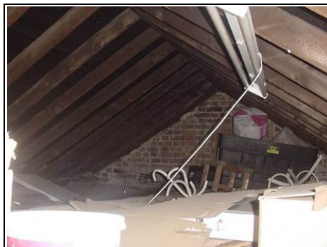
General view of the roof
