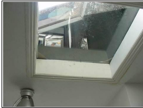
Access onto the roof
