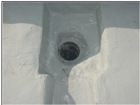
Acrylic paint has been painted over fixing holes for the leaf guard
