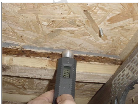
Reading 106 Against box guttering
