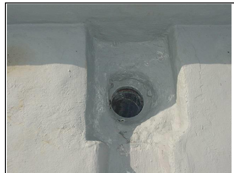
Box gutter to gulley point detail
