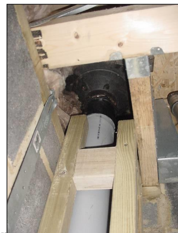
Outlet and the downpipe
