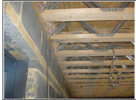
Joists forming support to roof decking
