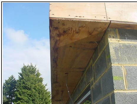
Fascia board to front
