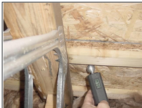
Reading 76 Base of box gutter
