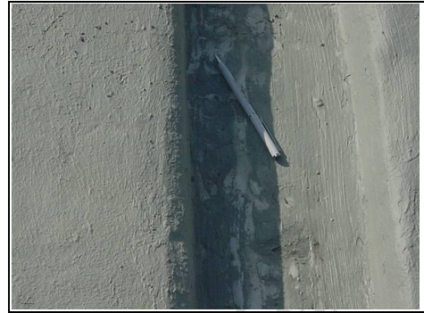
Close up of box gutter
