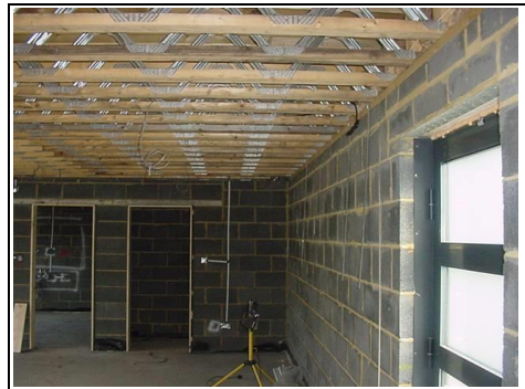
Blockwork walls support roof joists and decking
