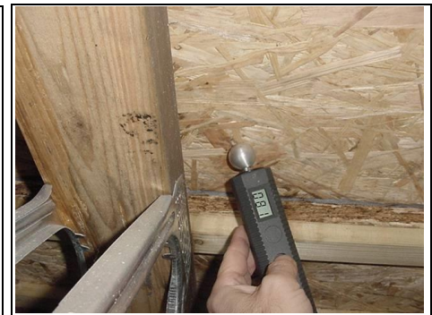
Reading 81 Area close to box gutter
