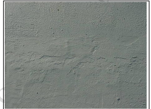
Close up of surface
