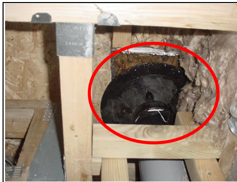
Outlet and gully within roof area
