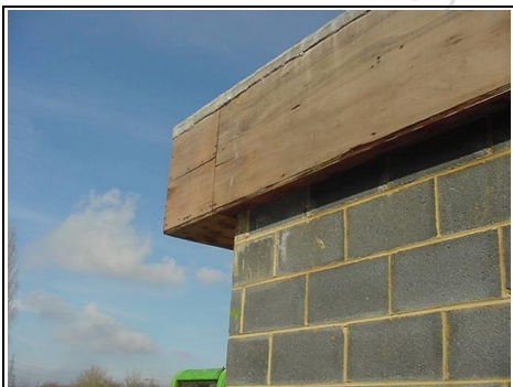
Fascia and soffit from ground level
