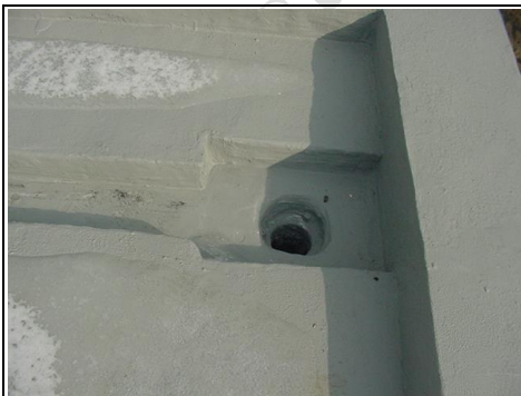
Gully from roof level
