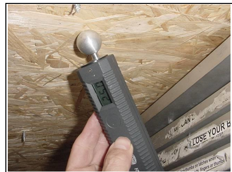
Reading 52 Away from box guttering
