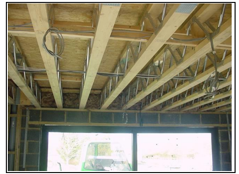
Underside of the roof
