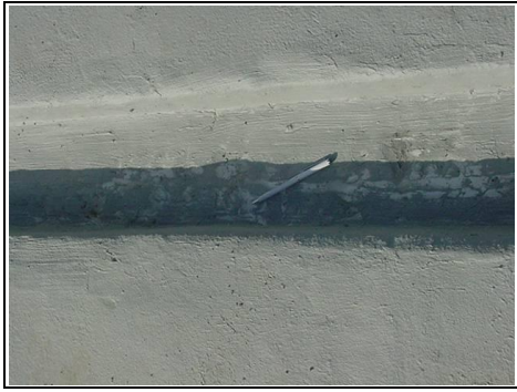
Marks within box gutter
